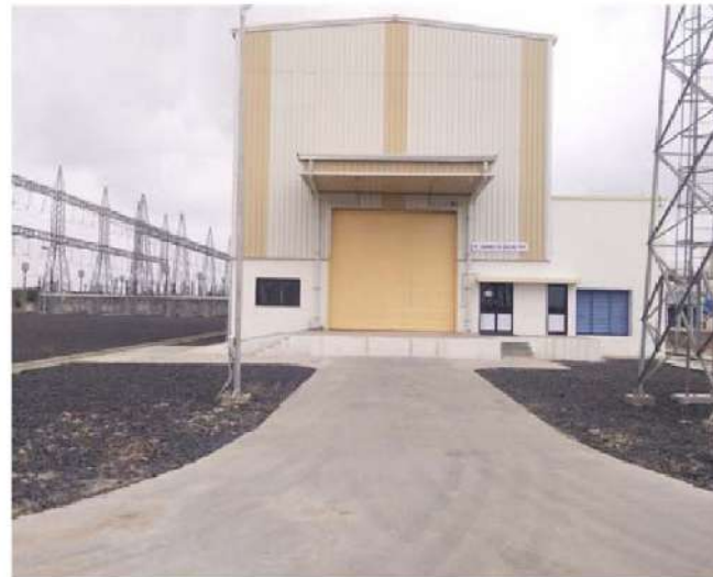
220KV GIS Building
