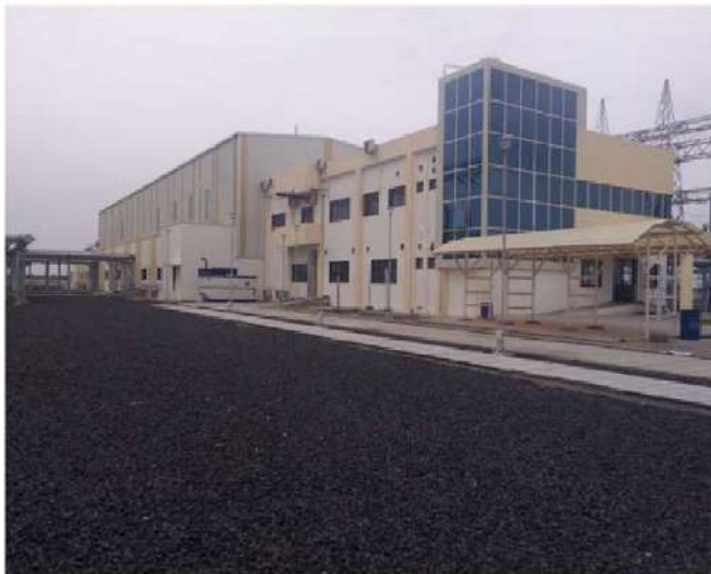
Control Room cum 400KV GIS Building
